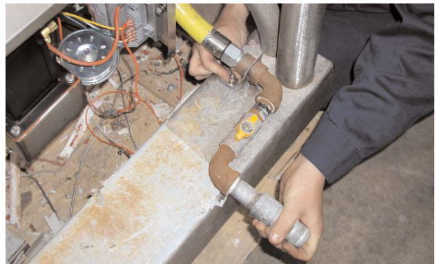
15. Fasten gas line bracket to back of frame (washers, lockwashers and nuts).
