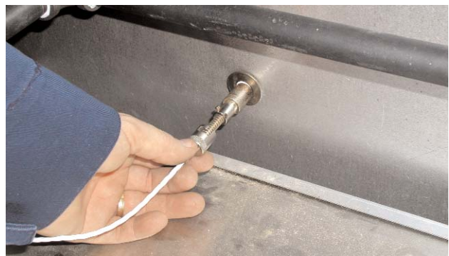
14. Insert operating thermostat.
