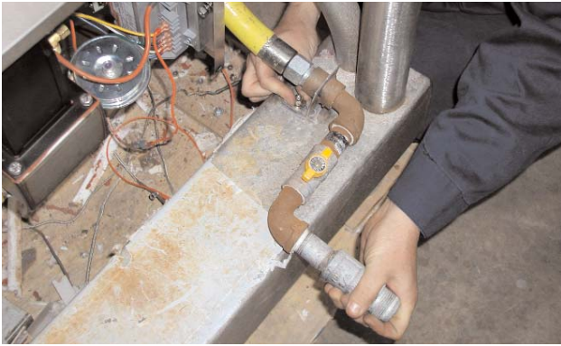
7. Remove gas line bracket.
