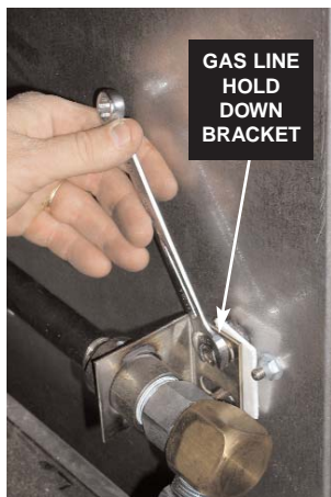
12. Place gas line mount gasket in position. Attach gas line hold down bracket.
