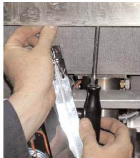
5. Remove safety thermostat cover, insulation and safety thermostat.
