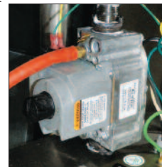
7. Gas Valve (showing hose for pressure tap)
