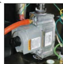
7. Gas Valve (showing hose for pressure tap)
