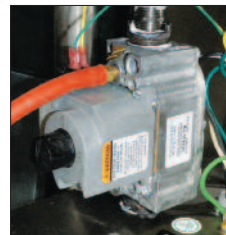
7. Gas Valve (showing hose for pressure tap)
