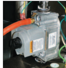
7. Gas Valve (showing hose for pressure tap)
