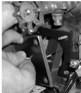
STEP 4 INSERT CLAMP BAR INTO BOILER HEATER HOLE WHILE RESTING BLOCK-OFF PLATE ON #6-32 SCREW.
