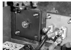
STEP 9 INSTALLATION COMPLETE. RECONNECT POWER AND CHECK FOR LEAKS. CAUTION: DISCONNECT POWER BEFORE TIGHTENING NUT IF LEAKS ARE PRESENT.
