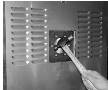
Figure 4 Cleaning the Inside of the Boiler Opening
