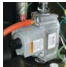
7. Gas Valve (showing hose for Pressure tap)
