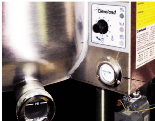
5. Kettle Jacket Water Sight Glass
