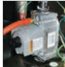
7. Gas Valve (showing hose for pressure tap)
